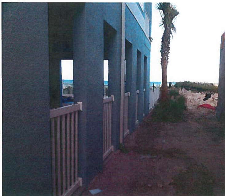
RIGHT SIDE (NORTH) VIEW 8/19/2015
