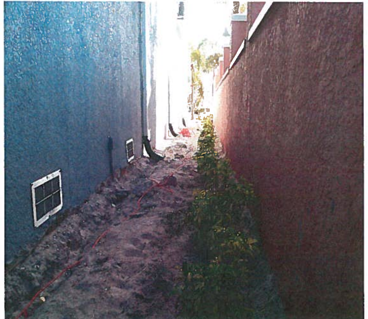
LEFT SIDE (SOUTH) VIEW 8/19/2015
